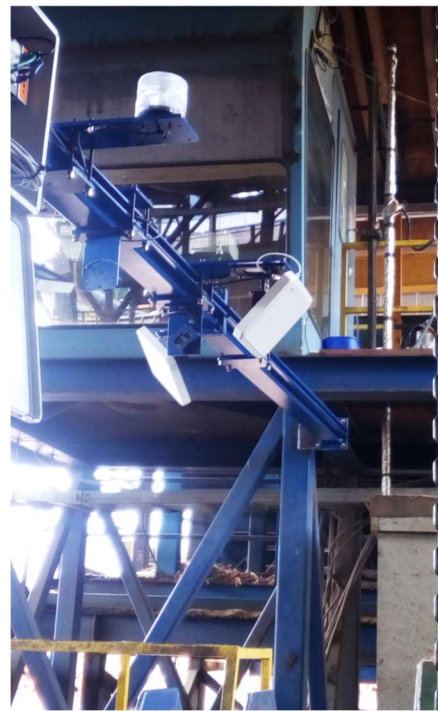
IBC Log Infeed RFID Portal 2
