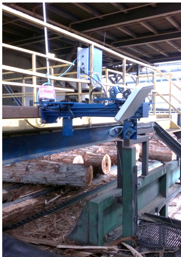
IBC Log Infeed RFID Portal
